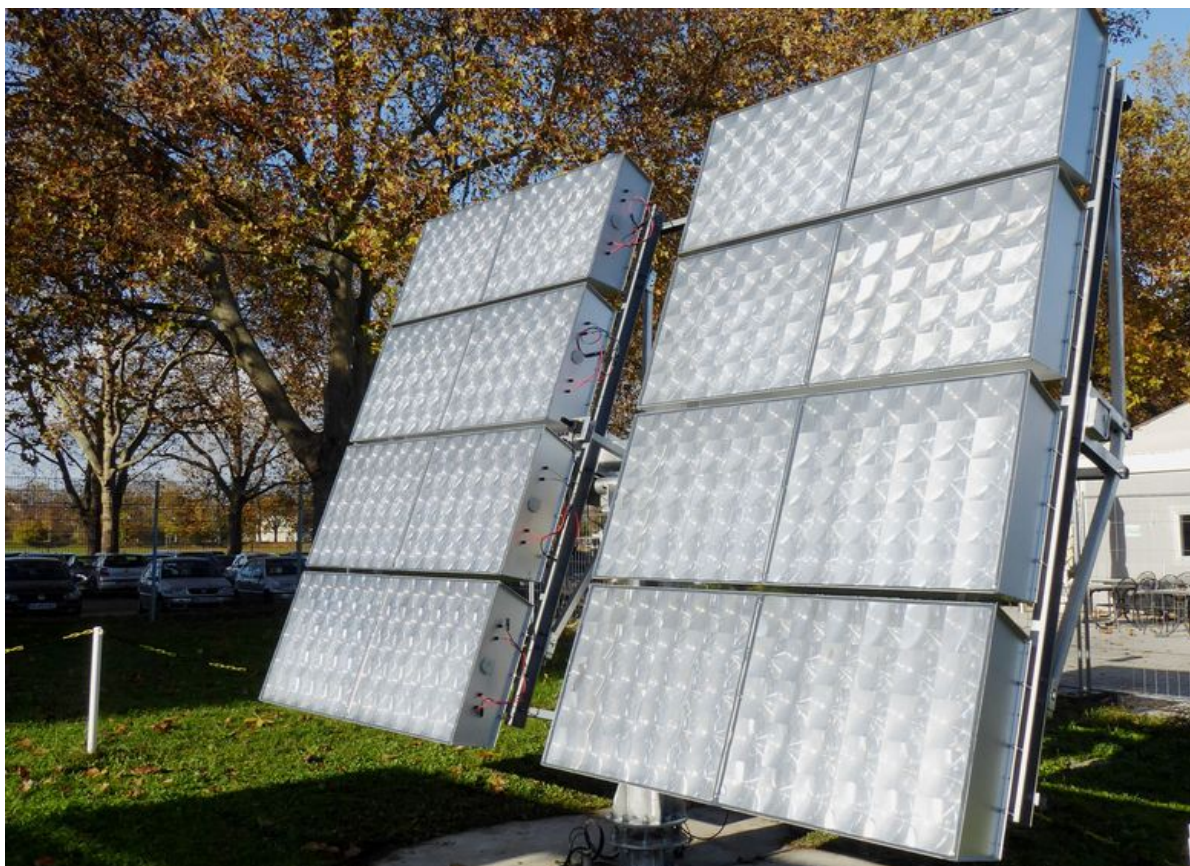
Concentrator photovoltaic modules fully installed on a dual-axis tracker in Heilbronn.
