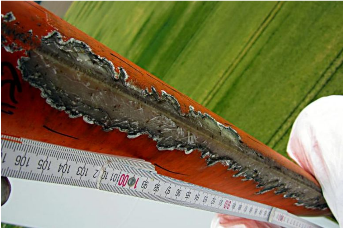
Damage to wind turbines, such as here on the leading edge of a rotor blade, requires extensive service work and the deployment of special personnel capable of working at height.
