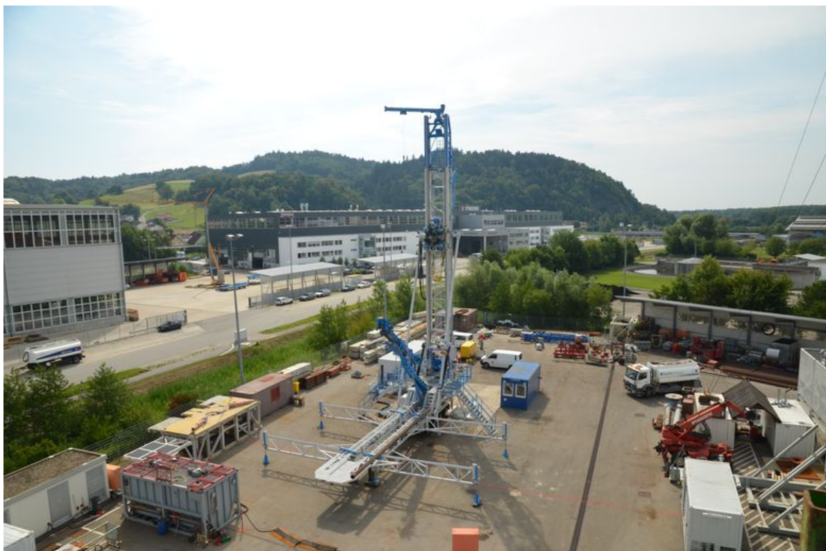
Workover rig set up for test operation
